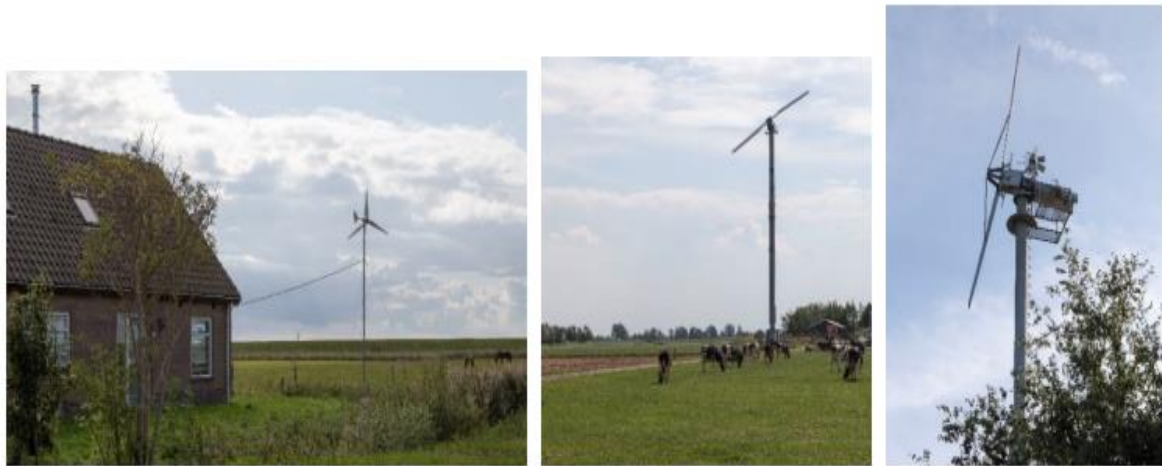
Figure 1. Examples of micro and small wind turbines in the Netherlands
